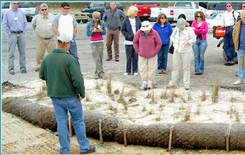
Stakeholders observe a shoreline restoration project that will create habitat and provide erosion protection without a seawall.
